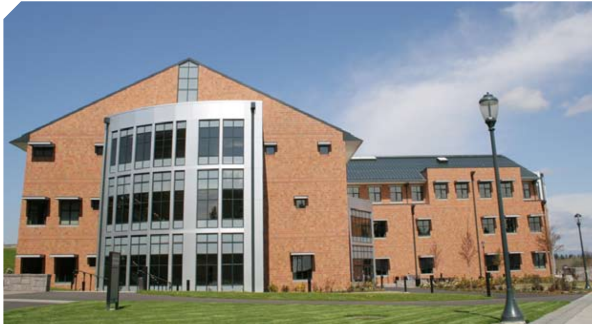
The Clark College at WSU-Vancouver facility, completed in spring 2006, opened up opportunities for students in north Clark County to attend Clark College classes closer to home and houses the college’s nursing program.
